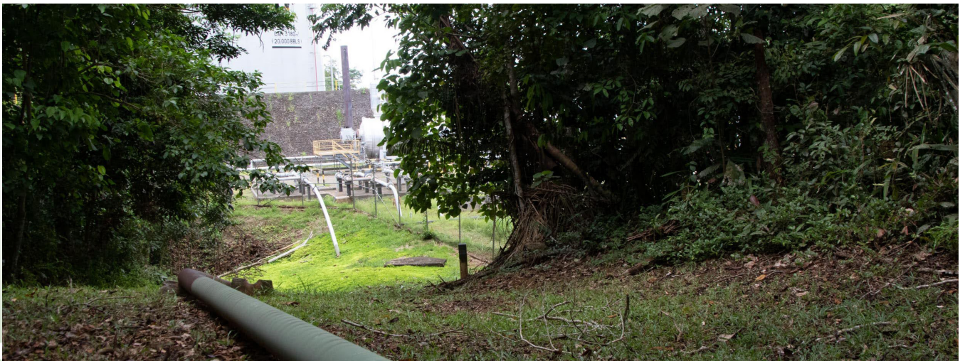
Oil well and transportation pipelines. Photo: Iván Castaneira/Tegantai Ecological News Agency
